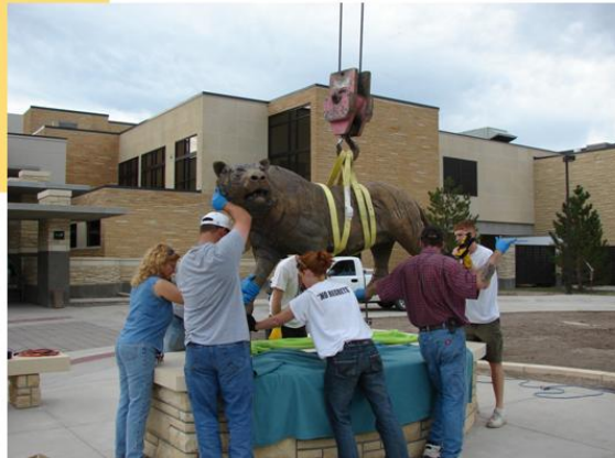
Memorial Union undergoing renovation
