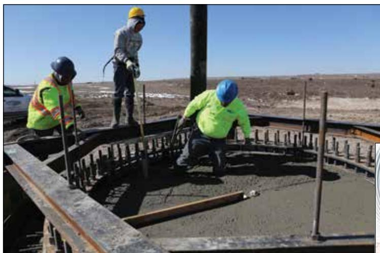
Workers for PNE Corp., Longview, Wash., left, completed the second of the two bases on March 5. The foundation is about 30 feet deep, below. The collar holds 128 inch-and-a-quarter bolts, which run 27 feet to the surface. Concrete is poured around the metal pipe, forming a long tube which is filled with uncompact excavation material, which is capped with concrete.
