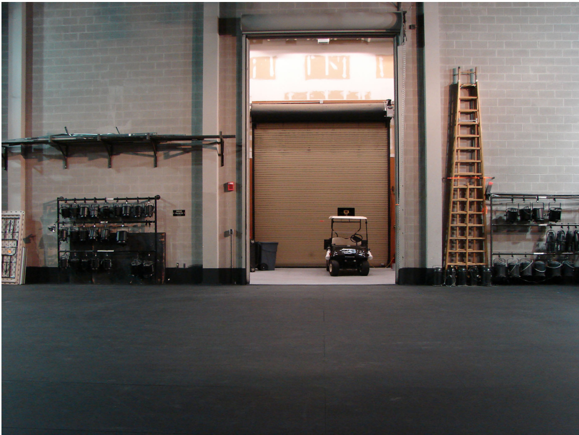
Interior and Exterior Loading Doors
